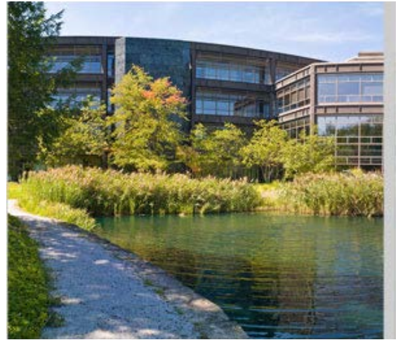
Cleveland Clinic's Lyndhurst Office Building was ENERGY STAR certified for the fourth consecutive year in 2013.
